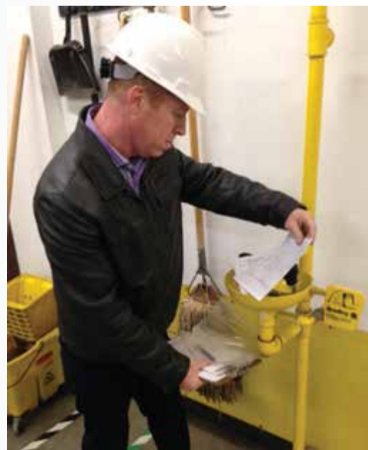
Mr. Tim Hahn, Ground Safety Specialist, reviews the inspection tag and serviceability of an emergency eye-wash shower during a unit annual inspection.
